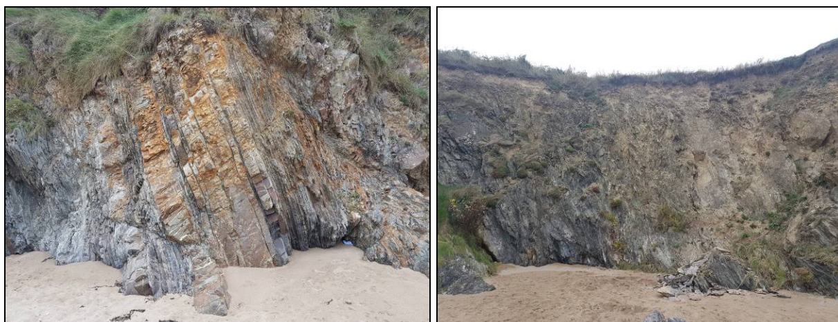
Plate 6 – Cliff rock strata and cliff (left) and the cliff on the cable route (right)
